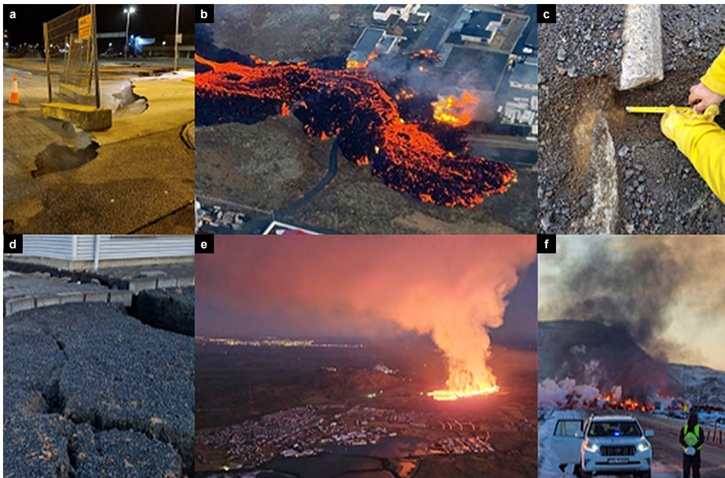
Figure 1 a) Main graben fault through centre of Grindavík; b) the only lava flow to enter Grindavík during this eruptive period (14 January 2024, Hólmfríður Dagný/ruv.is); c) evidence of strike-slip movement on faults cutting the town; d) damage to building foundations; e) January 2024 eruptive fissure outside of Grindavík town (Björn Oddsson/ Civil Protection); f) lava cuts the main road to Grindavík, Svartsengi powerplant, and the Blue Lagoon.
