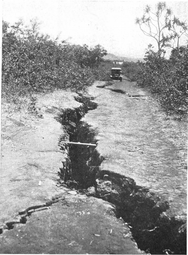
FIG. 2.—Cracks two feet wide, looking southwest toward Kapoho village. About April 24, 1924. Photo by Tai Sing Loo.
